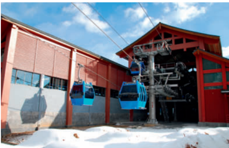
The lower station seen from the line, with the parking shed on the left. Above the 8-seater gondola one can again see the evacuation ropeway, with the second rescue car above a Sigma gondola in the middle of the photo.
