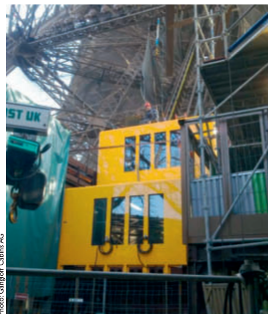
Gangloff's engineers installing the elevator cars on the west leg of the Eiffel Tower
