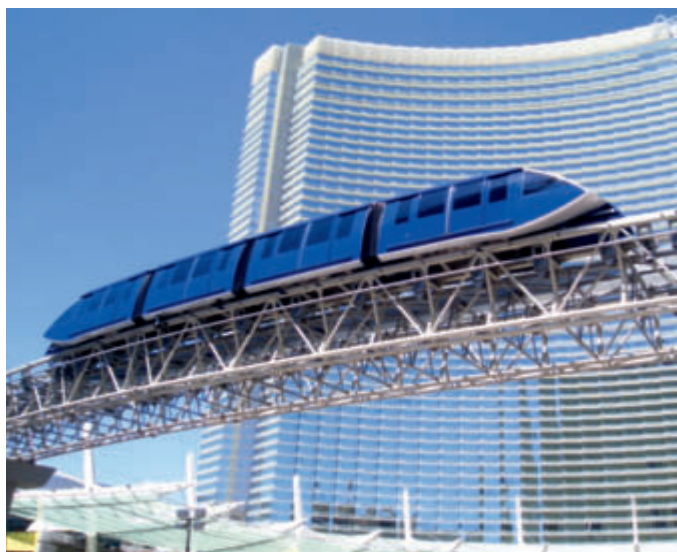
The DCC Cable Liner in front of the huge MGM CityCenter complex
