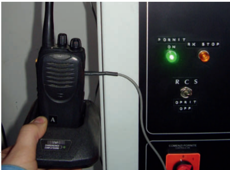
The radio station and its control buttons from the main cabinet in the control room
